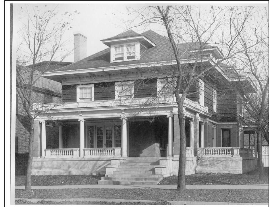
The Rohrbaugh Home north of the Church
