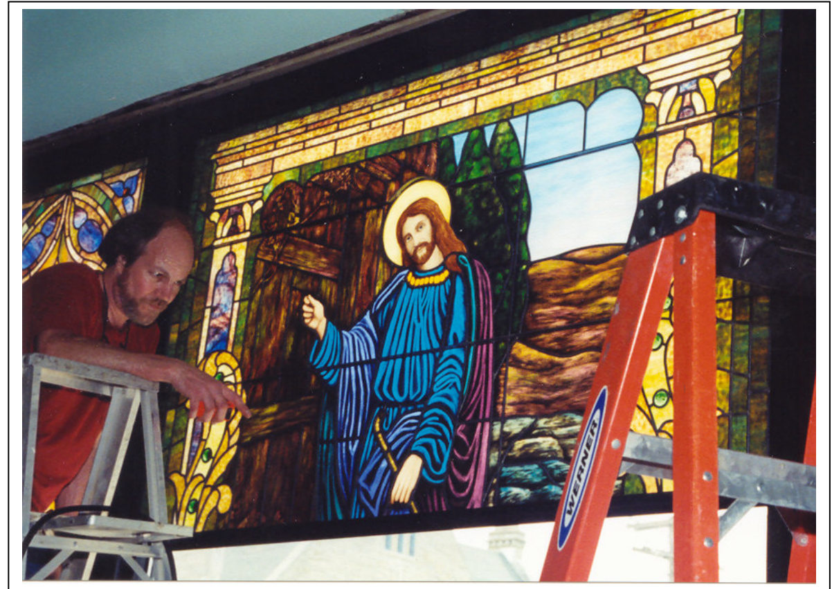
Cliff Mayfield of Karen Hendrix & Associates installing the replacement “Jesus Knocking” stained glass window.
